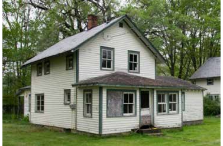
5/13/2016 - Condition before repairs
