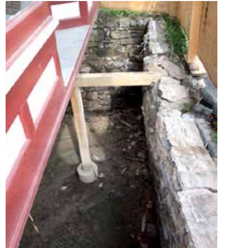
Photo A - Newer support beams, under the front porch
